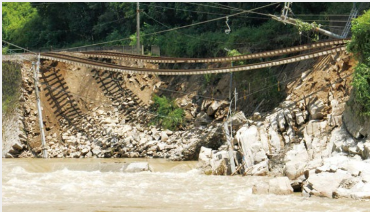
Damaged Railway by torrential rain in July, 2018 in Higashihiroshima city
