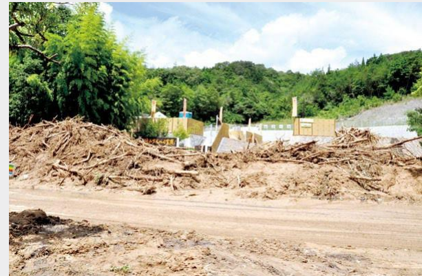
Landslide by torrential rain in July, 2018 near the Higashihiroshima campus
